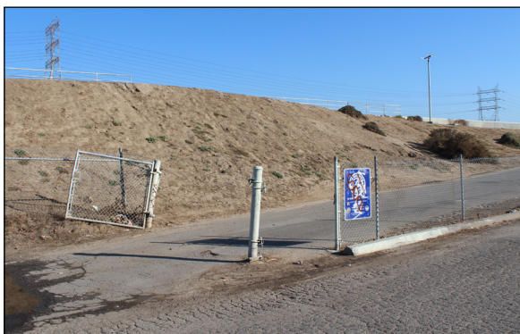
The entrance to the Los Angeles River Bikeway at Tweedy Boulevard is unmarked and poorly maintained. It provides a significant opportunity to improve physical conditions, and provide amenities and directional signage.
