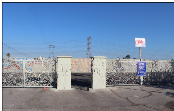
While the entrance to the Los Angeles River Bike Path at Southern Avenue has a decorative entrance, it is also in need of improvements.
