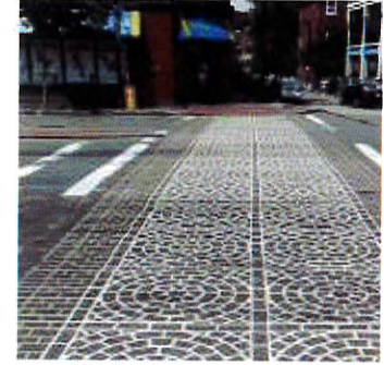
ENHANCED CROSSWALK THERMOPLASTIC
