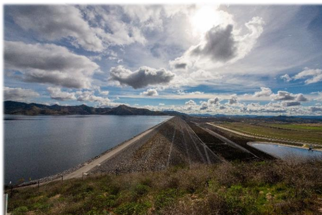
Figure 4: MWD's Diamond Valley Lake (Potential Reserves for WSAP Allocations)
