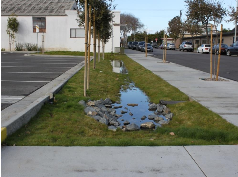
Figure 2: Vegetated Swale (Signal Hill, CA).
