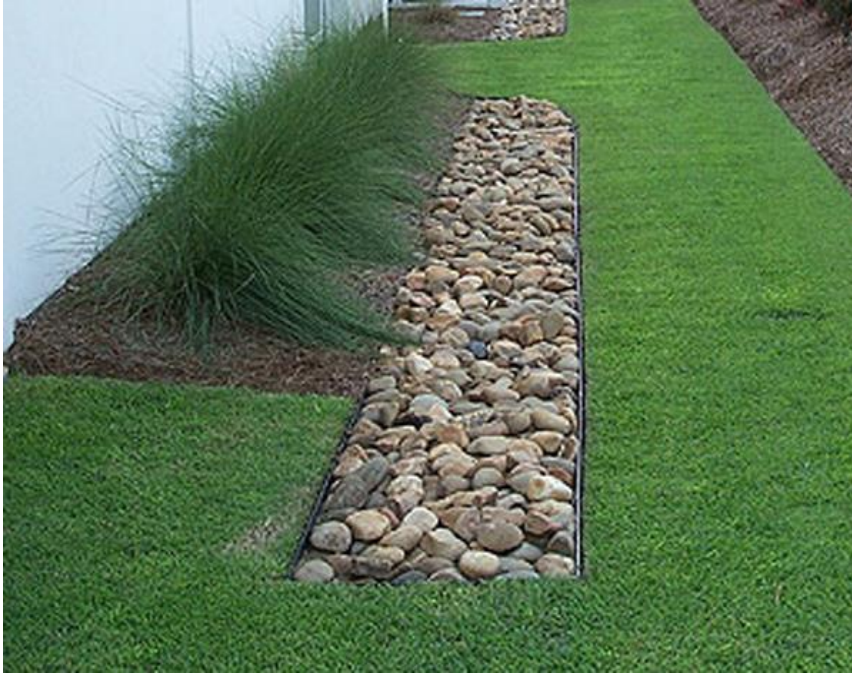
Figure 5: Infiltration trench ( http://www.cob.org/services/environment/water-quality/ ).
