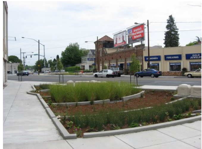
Figure 2. This bioretention area takes runoff from the street through a trench drain in the sidewalk as well as runoff from the sidewalk through curb cuts (Source: Abby Hall, US EPA).
