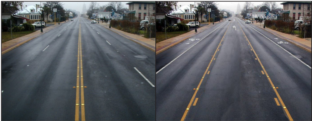
Figure 9-30: Before and After Road Diet
