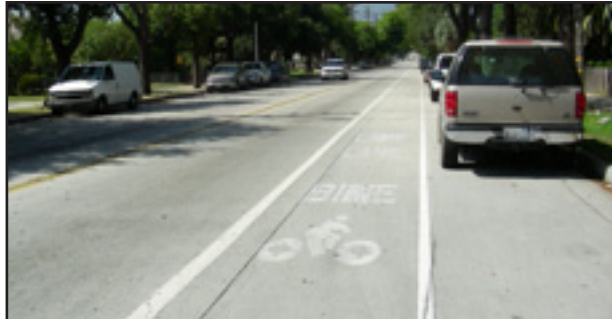
Figure 9-3: Bike Lane Striping and Stencil
