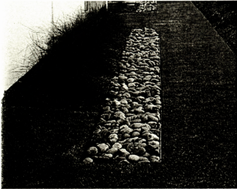
Figure 5: Infiltration trench ( http://www.cob.org/services/environment/water-quality/ ).
