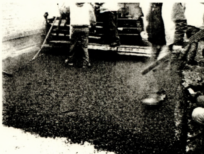
Figure 9: Permeable Asphalt Installation Using Ground Tire Rubber.
