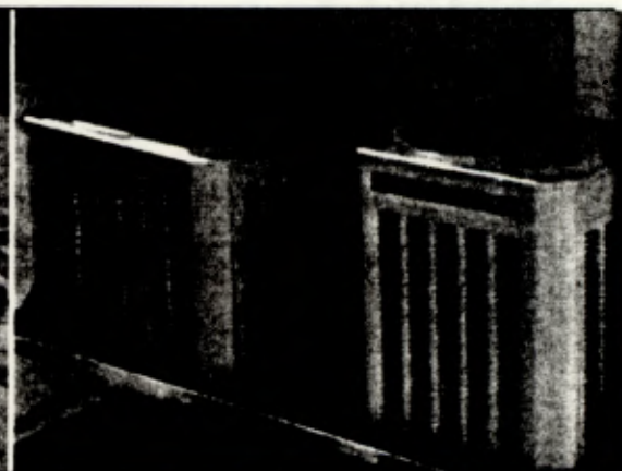
Package units serving areas not served by CHW system
