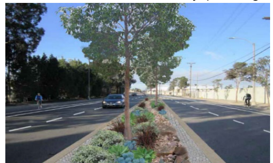
Garfield Ave and Imperial Hwy Street Improvements
