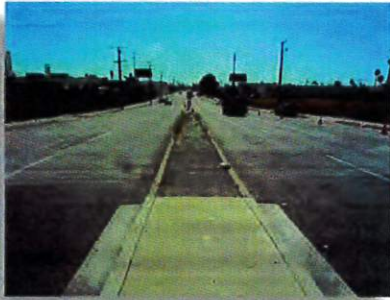
Existing Imperial Median
