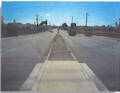
Existing Imperial Median
