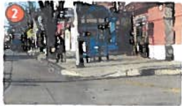
All non-ADA compliant ramps to be updated.
