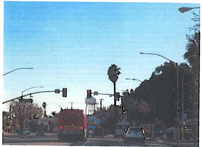
Long Beach Boulevard Existing Conditions
