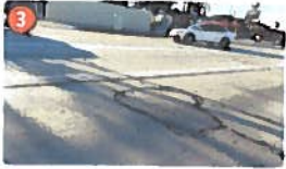
Cost-efficient pavement strategies will be formulated to rehabilitate the roadway surface.
