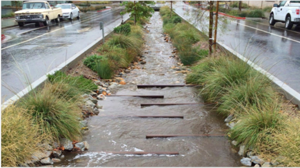
21st Street, Paso Robles, CA. Bioswale treatment of roadway runoff improves water quality.
