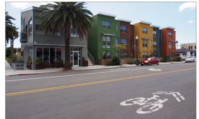
North Park, CA. Sharrows provide mixed vehicular and bicycle access within the primary road ROW.
